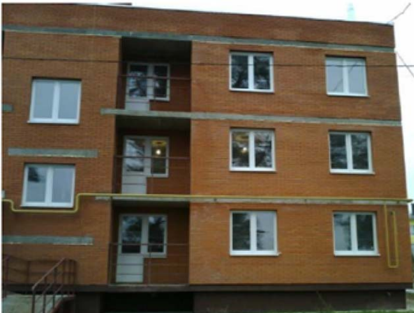
Fig. 6. The wall of the residential building under study with translucent structures.
